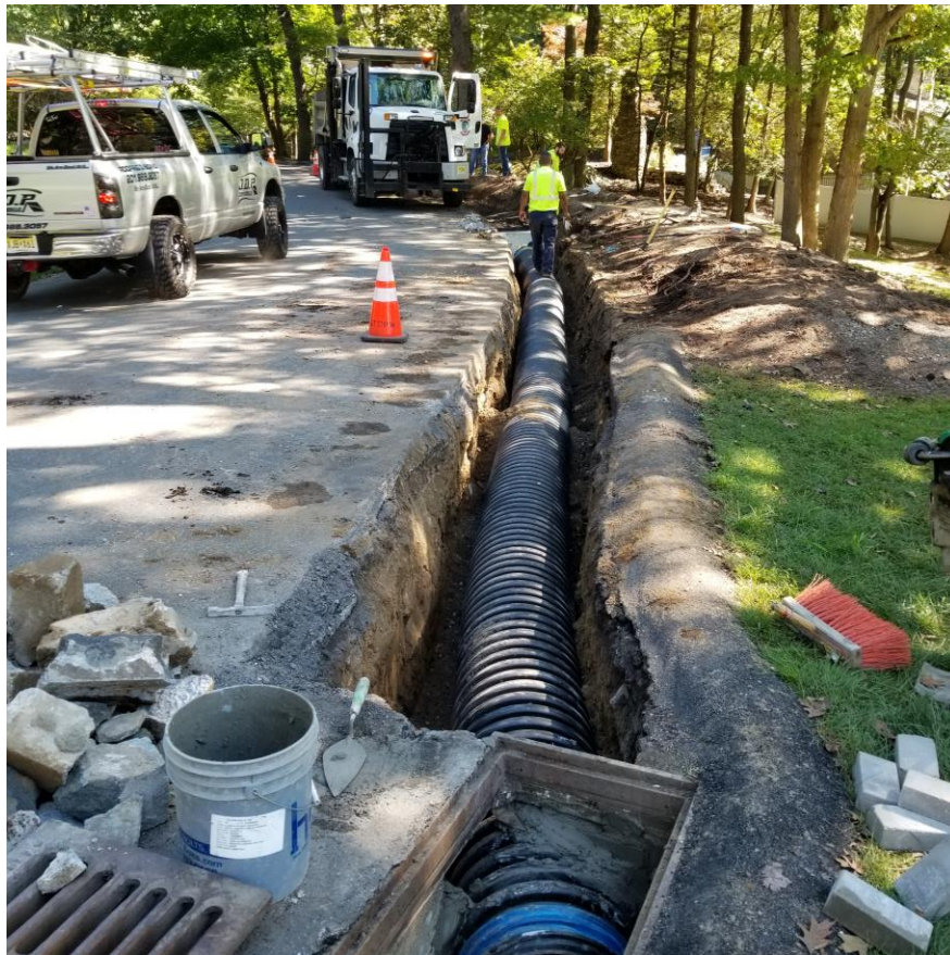
Figure 8: Stormwater Pipe Installed along Fox Hollow Road
